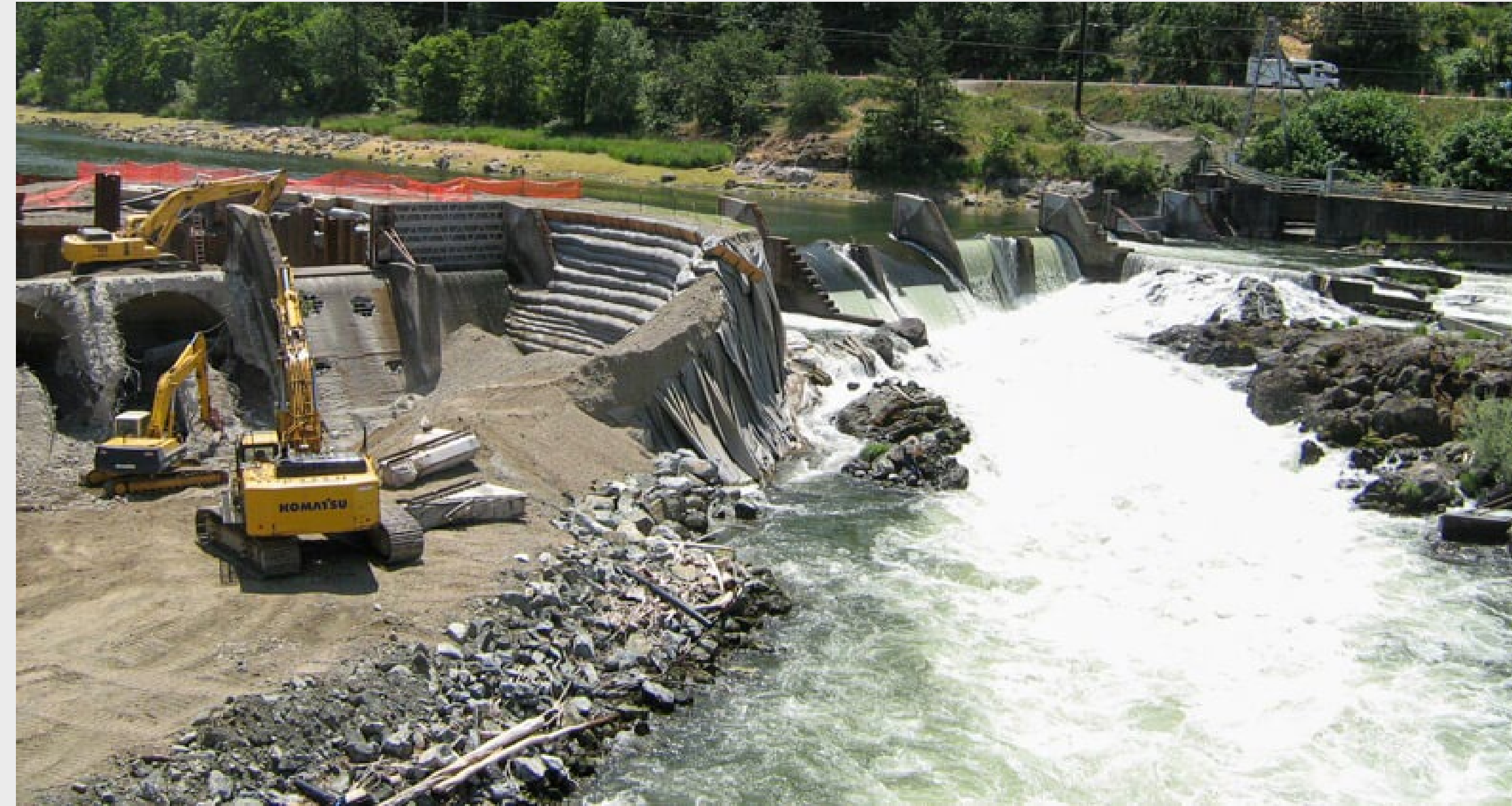
Savage Rapids Dam Removal (Northwest Demolition and Dismantling)
