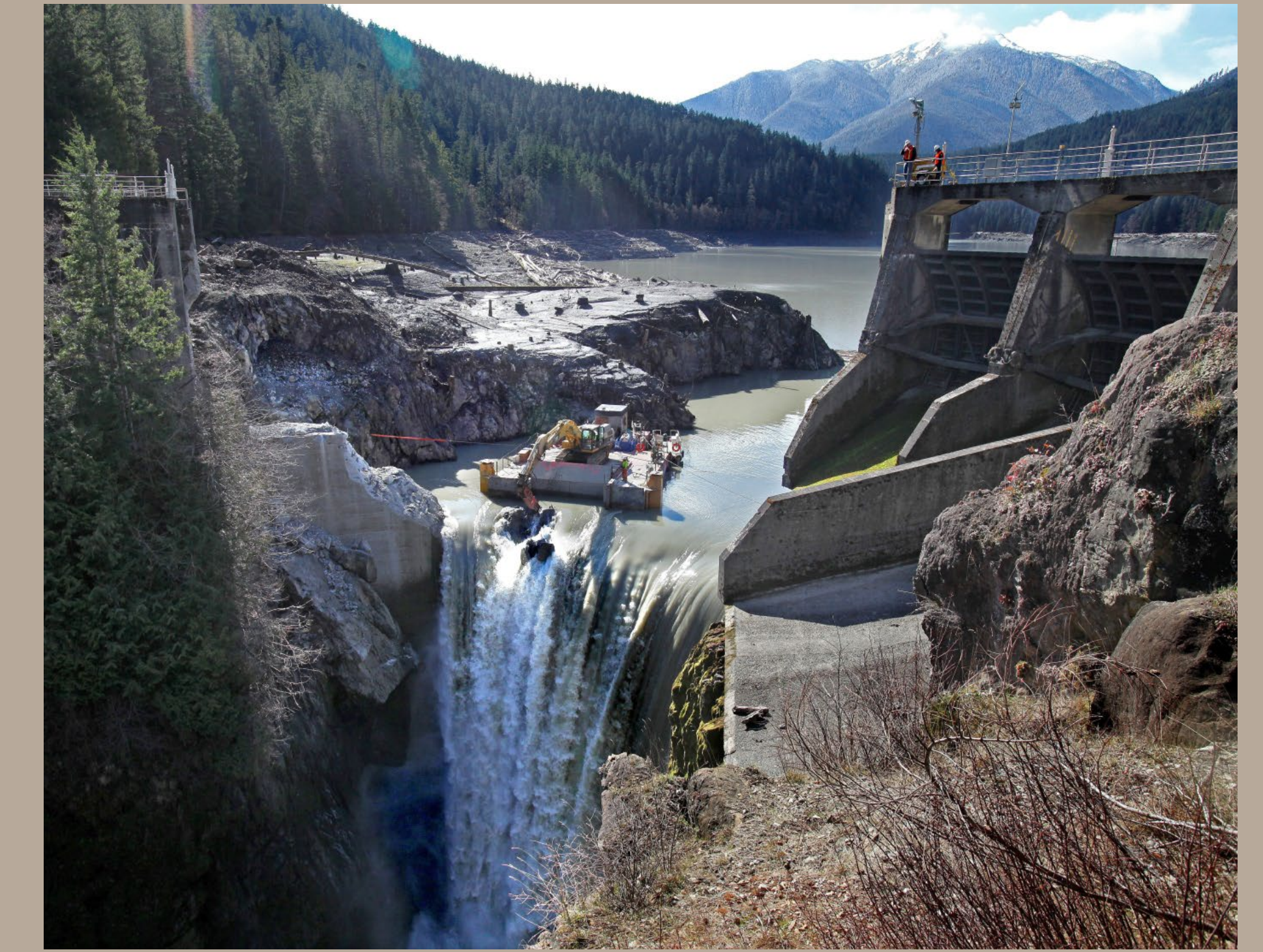
Elwha Dam Removal (AP Photo/The Seattle Times, Steve Ringman)
