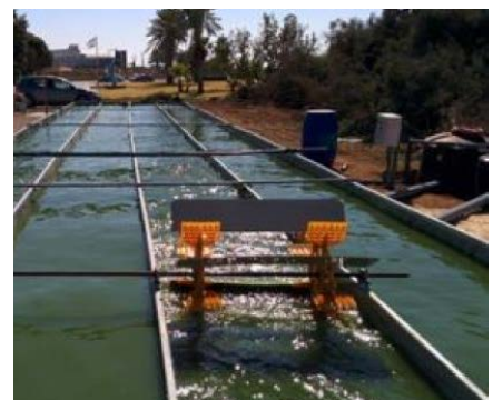
Wastewater treatment using algae. This plant is part of a startup company using this process in developing countries to provide clean water and save energy.
