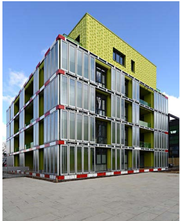
The Bio Intelligent Quotient, is an apartment building in Hamburg, Germany. Algae-powered energy technologies heat the water and air in the building. Source: New York Times 5 .
