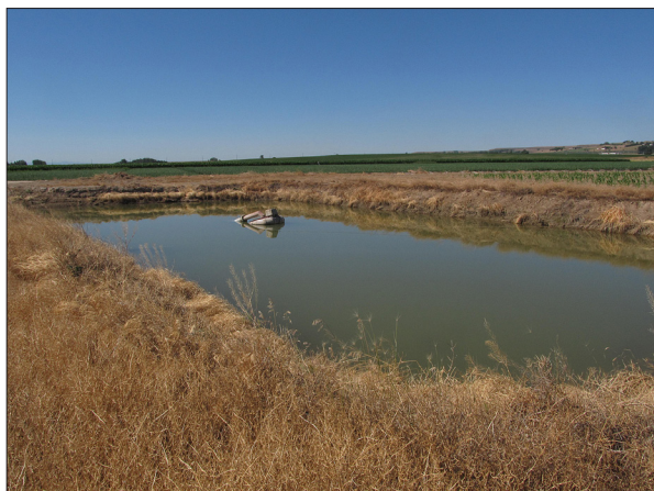
Figure 4. A sedimentation pond that utilizes a pumpback system to return runoff water to the field.
