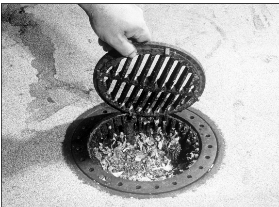
Figure 5. Don't forget the drains — they can be a source of bad odors. Cleaning is not finished until the drains are cleaned.
