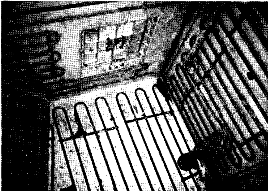
Figure 2-7. Arrangement of Coils in Fish Well
